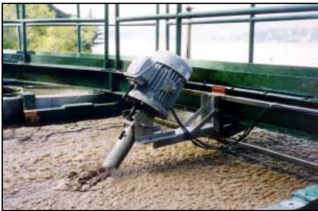
Typical TORNADO Aerator Installation.
