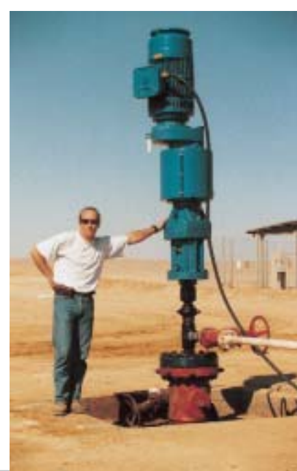
Commissioning a PCP in Libya (Drivehead VS 60 HP with moto-reducer)
