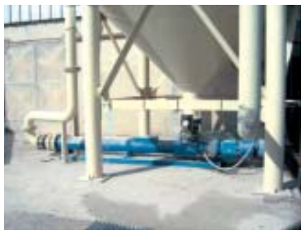
I pump for filter press feeding in minerals application
